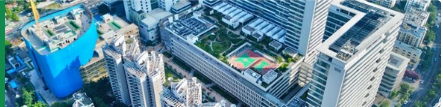
Expansion project photograph • Online source: China State Construction
